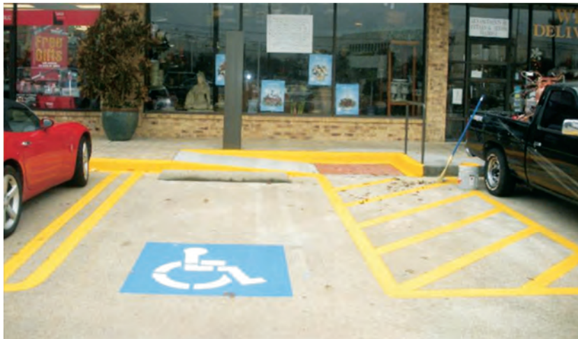
Photo 16 Accessible Parking with Aisle Space and Kerb Ramp
