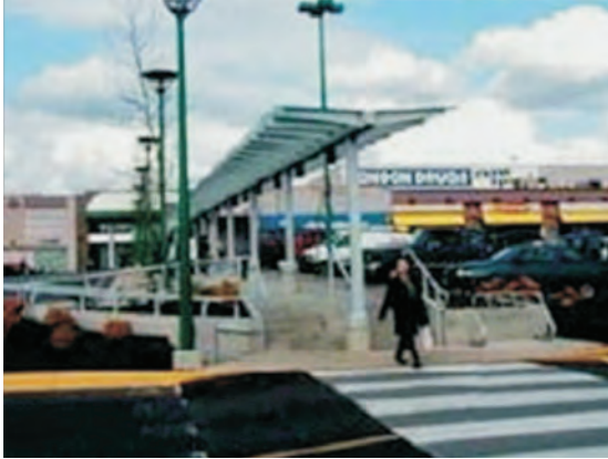
Photo 18 Pedestrian Facilities at Transit Area
