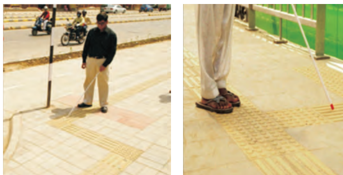
Photo 3 Configuration of Floor Tactile Paving
