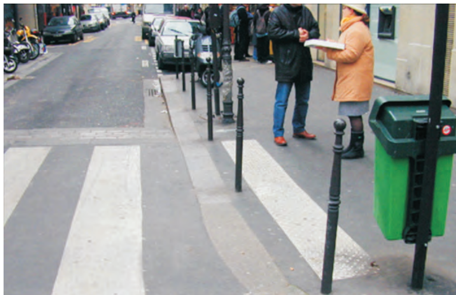
Photo 7 Raised Pedestrian Crossings (Table Top)
