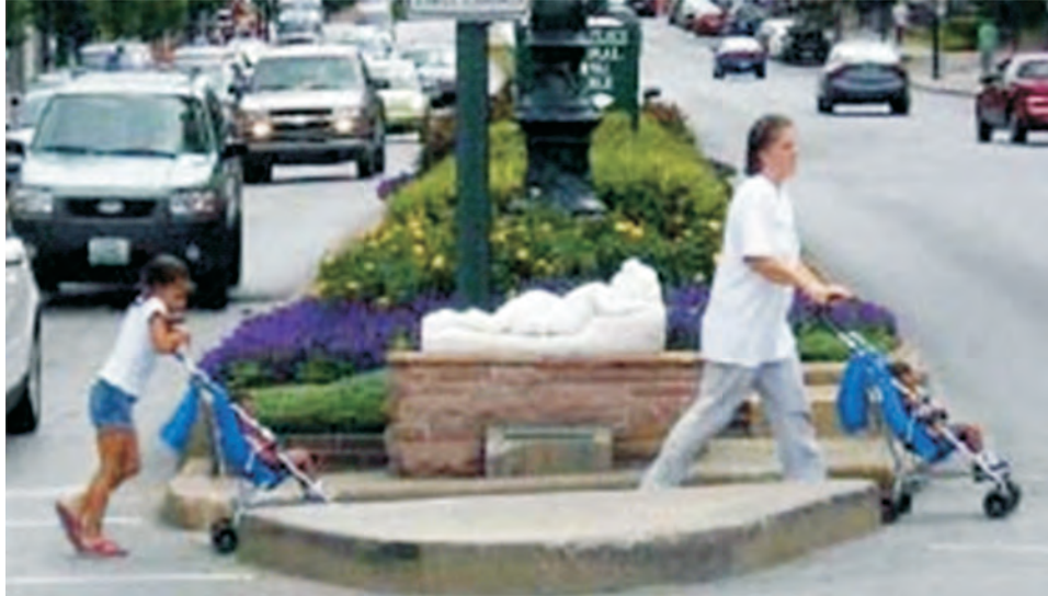
Photo 8 Median Pedestrian Refuge on Two-Way Road
