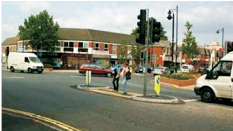
Photo 9 Median Pedestrian Refuge at Signal-Controlled Junction
